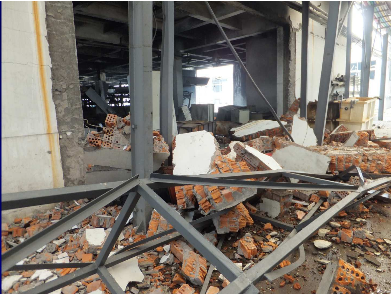
Figure 7-59. Collapsed and destroyed eastern wall and air conditioner. From Li et al. (2016)
