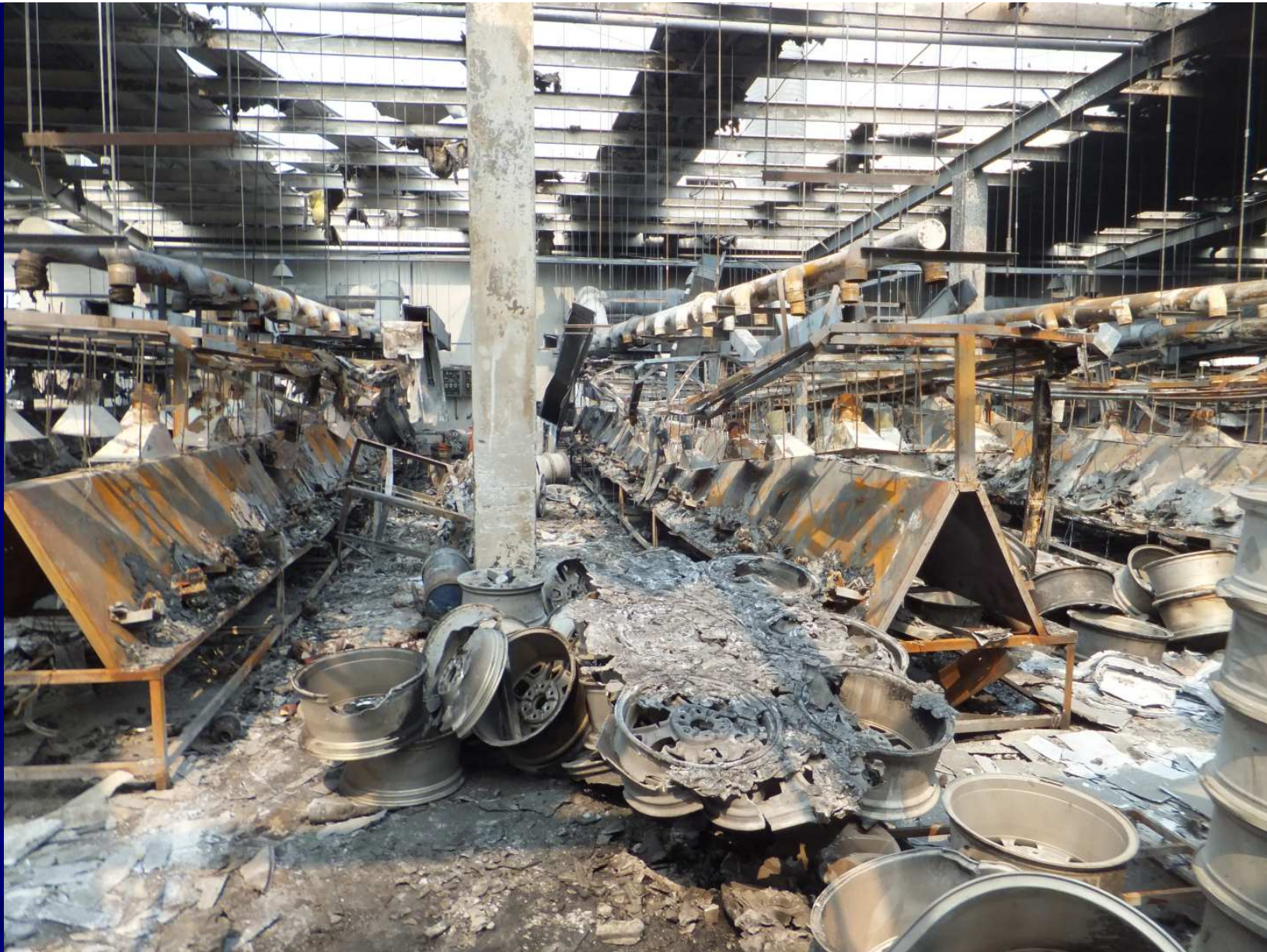
Figure 7-60. Destroyed process lines on the second floor. From Li et al. (2016)
