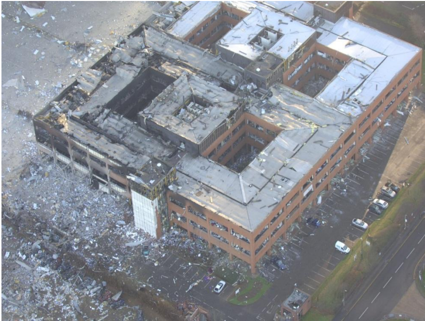
Buncefield, 11 December 2005, Northgate building
