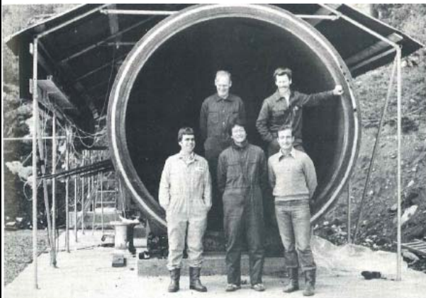
Flame acceleration experiments in 10-m 3 pipe, Raufoss, Norway, ~1980
